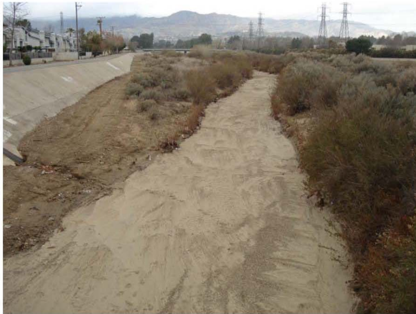
Stream Bed and Proposed Location of Rubber Dam No. 1 (Looking Downstream)
