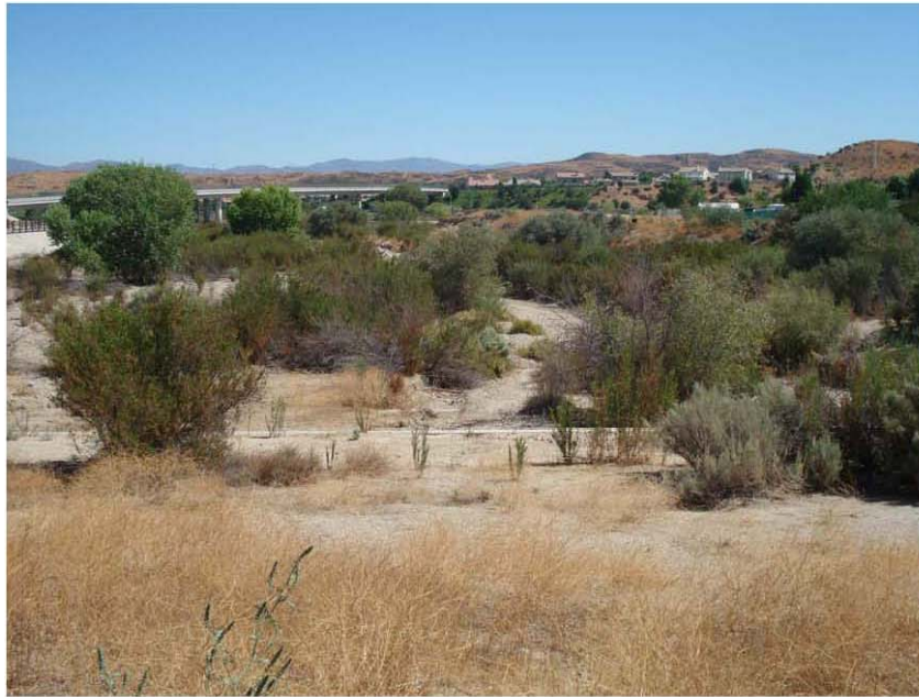
Existing Drop Structure at Rubber Dam Location No. 1 (Looking Upstream)
