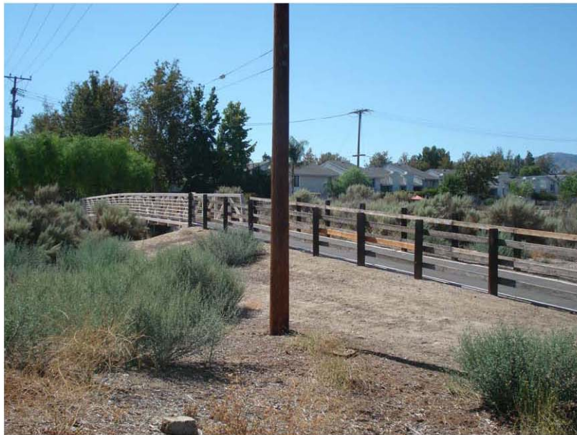
Pedestrian Bridge and Bike Trail at Dam Location No. 1 (Looking Downstream)
