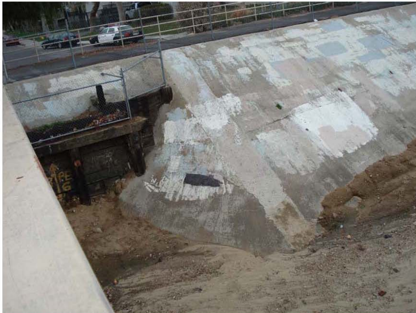
East Side Slopes Downstream of the Pedestrian Bridge (Looking Downstream)
